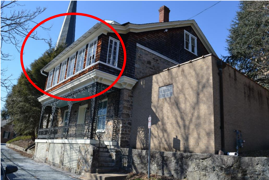
Figure 11 – Photo from application - enclosed area and roof extension proposed to be removed.
