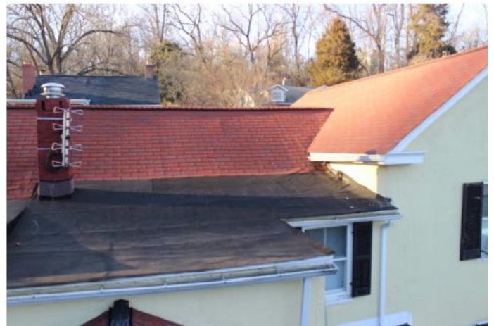
Figure 3 - Photo 4 from application showing flat roof to be raised.
