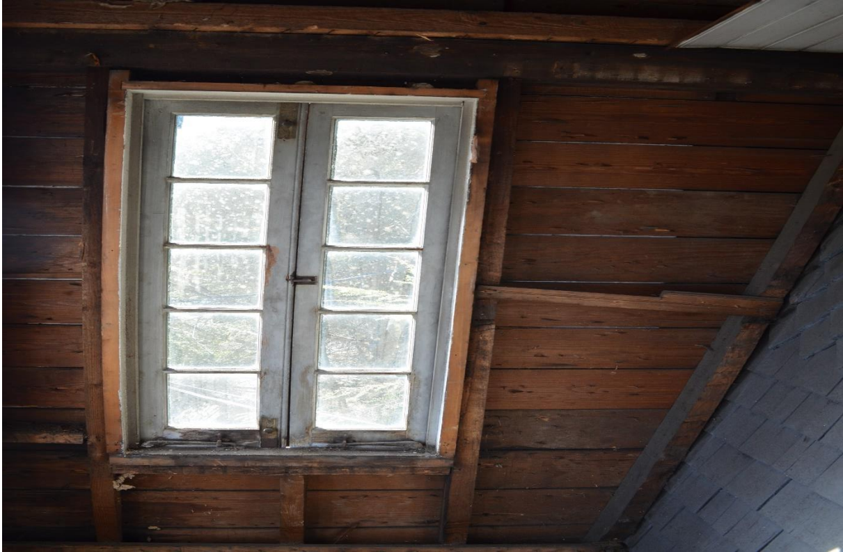
Figure 13 – Photo from application - Side wall to be removed where attached to shingle roof. End windows showing how the porch enclosure was added.
