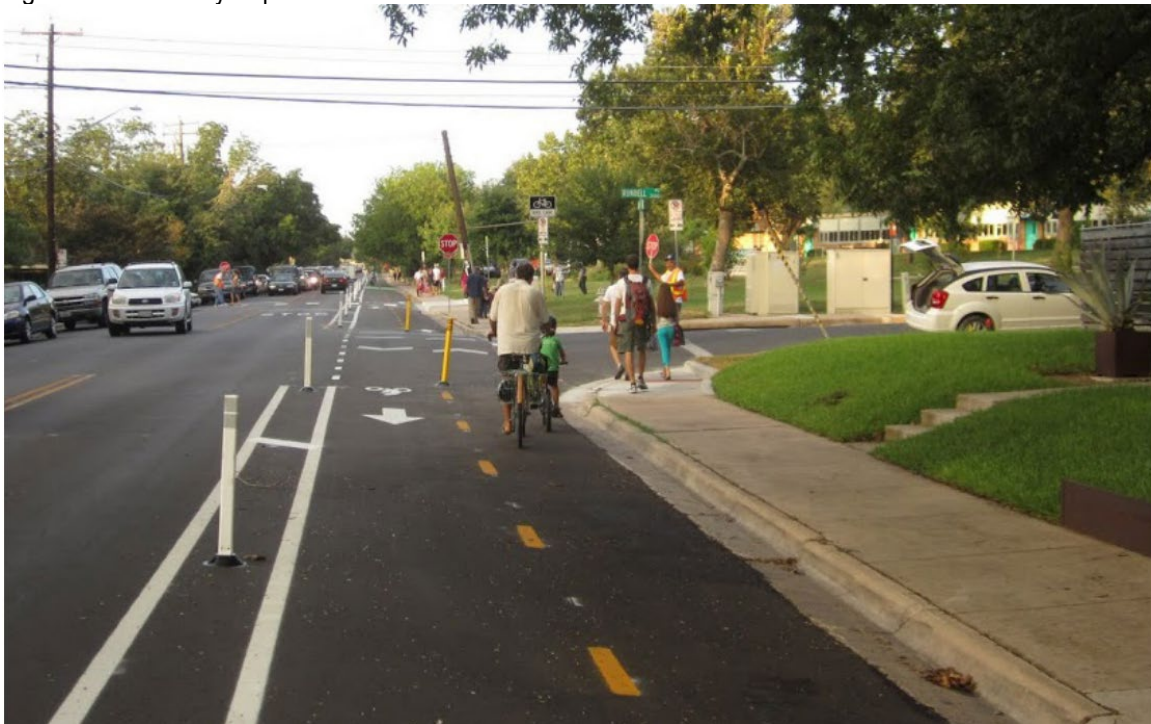
Figure 2-5. Two-Way Separated Bike Lane.
