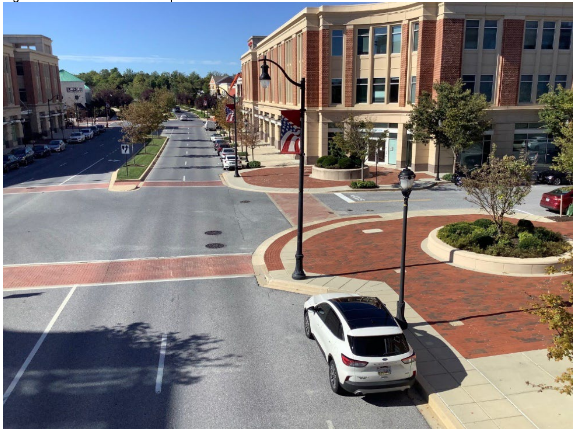
Figure 2-20. Mountable Truck Apron.
